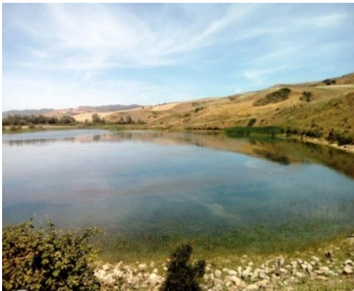
Fig. 9: Photo of the Gares Rouiba hillside reservoir. (2017).
