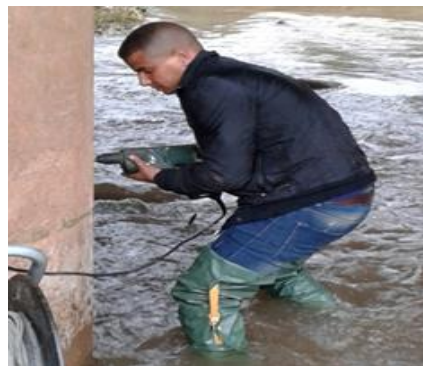
Photo sheets 1: installation and monitoring of the limnimétrique scale
